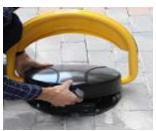
3. Use a pen to mark the three holes to confirm drilling positions.
